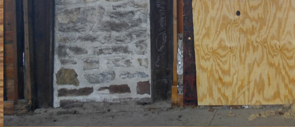
Missing freight doors with broken framing
