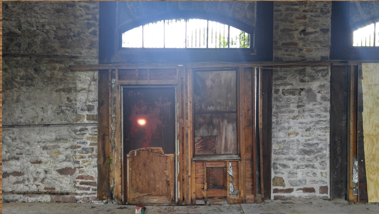
Missing freight doors with broken framing
