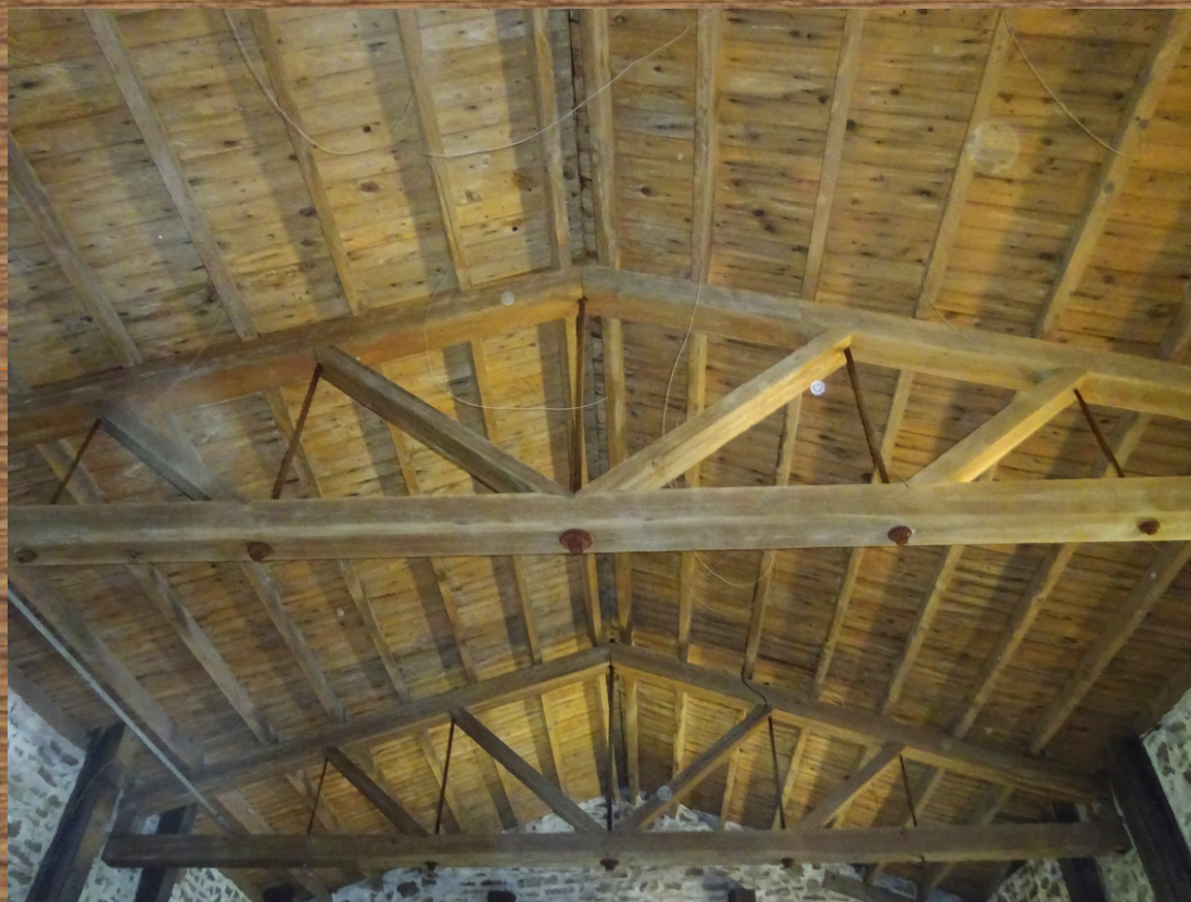
Original ceiling rafters and roof joists
